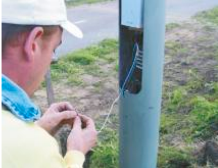
NivuChannel power supply using the street lighting
