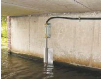
Installed rod sensor with accessories
