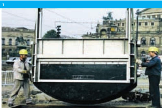
1 Regulating gate and sluice gate combination front side, installed in the sewer system of Dresden, Germany
